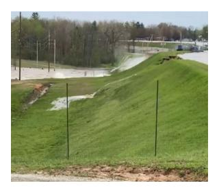
196. The embankment then rapidly collapsed in a landslide:
