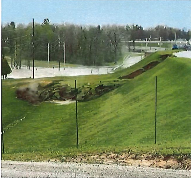
168. The full breach of the Edenville Dam followed within seconds:
